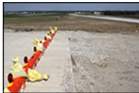
Airport construction to take off
